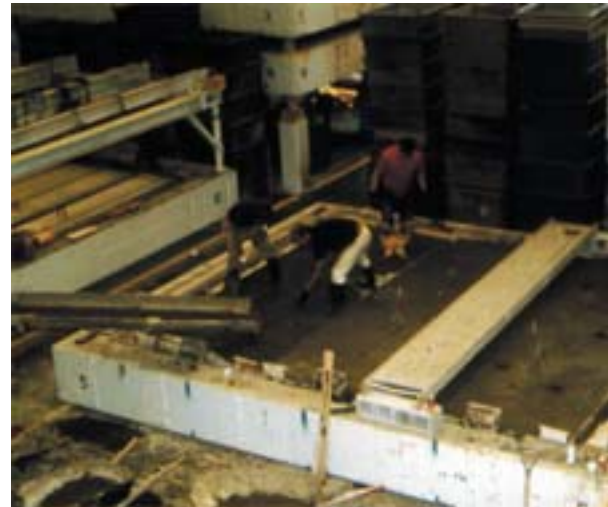
Photo 1. Workers construct sample building assemblies before testing can begin.
